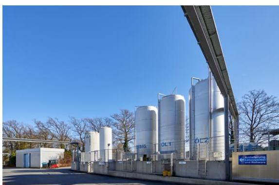
**Figure 4** - The tanks for cooking oil and vinegar are automatically filled by the respective suppliers three times a day
