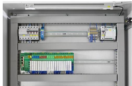
Figure 2 - ILC 2050 BI IoT-based controllers forward the acquired data to the Emylitycs building management system
