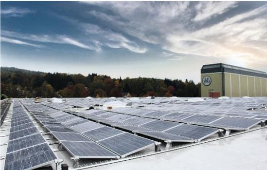
**Picture caption:** A factory roof at the works in Wiehl accommodates a 3,100-sqm photovoltaic system. (Photograph: BPW Bergische Achsen KG)
